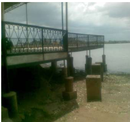
Songwa Club Office Balcony protruded into the Dam
